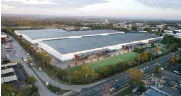
Forrester Distribution Centre
