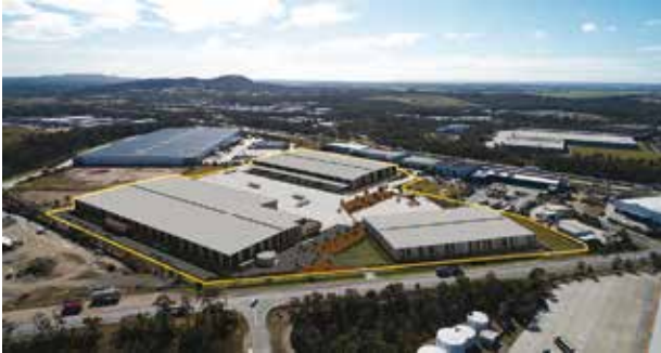
Yatala Distribution Centre
