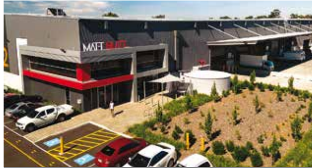
Oakleigh Industrial Estate
