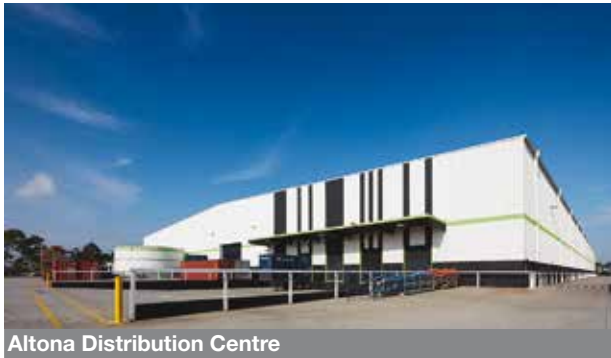
Altona Distribution Centre
