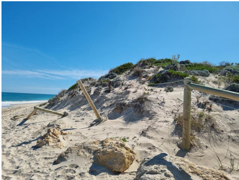
Plate 1: Photograph of undermined footings of fence at beach
