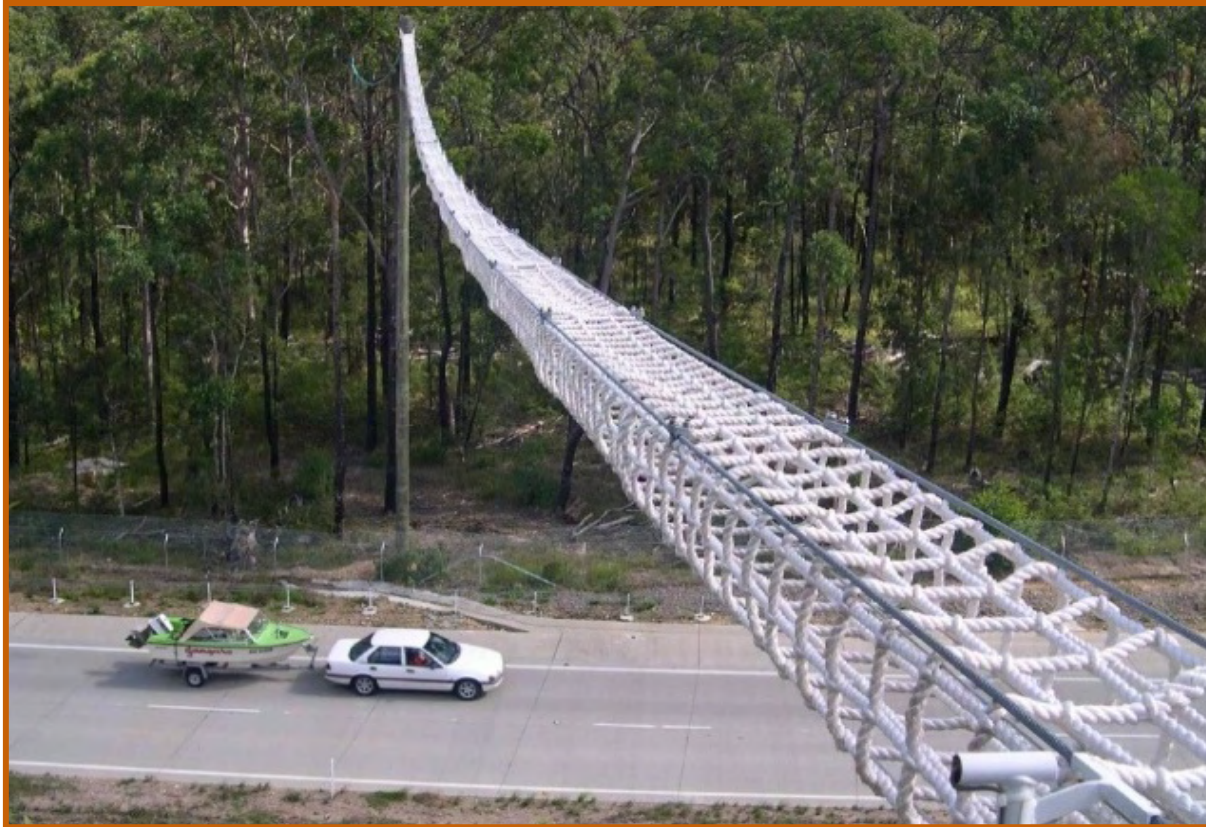
Photograph 1: Aerial fauna crossing in the Karuah Bypass on the Pacific Highway (Photos courtesy of David Bax, [Thiess Pty Ltd] 2006).
