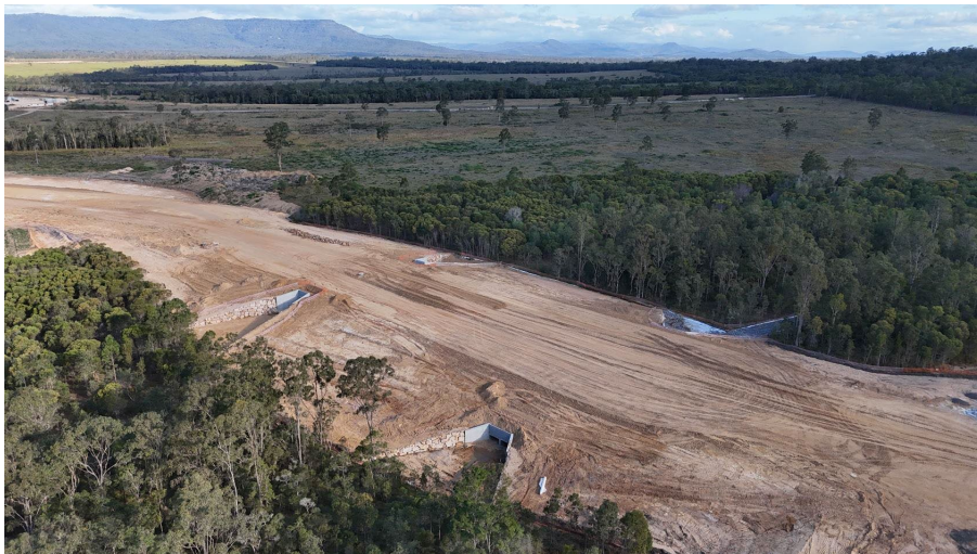
Culverts Structures Installed September 2024 (fauna culvert on left)
