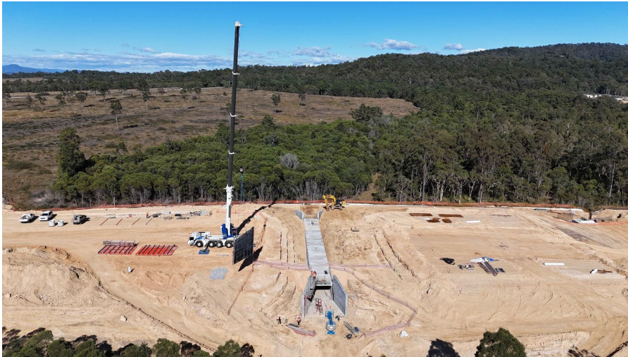
Fauna Culvert installation June 2024
