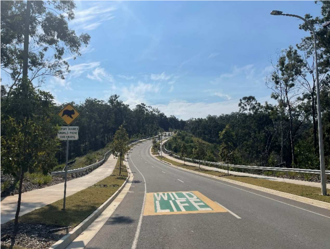
Photo 1: Fauna sensitive design including road markings and Koala awareness signage.
