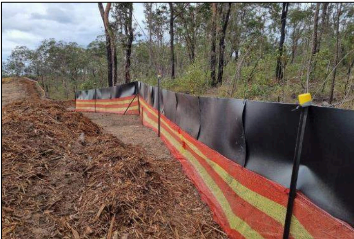
Photo 1: Temporary perimeter fauna exclusion fencing
