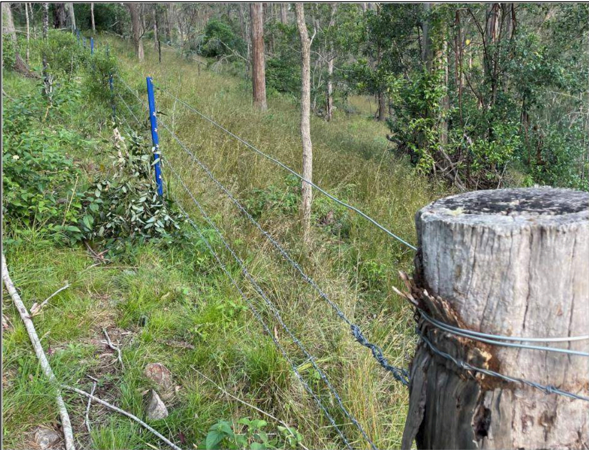
Photo set 3: After photos – Perimeter fence with top strand of plain wire
