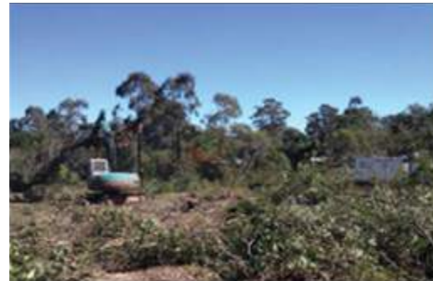
Photo: Control clearing of vegetation
