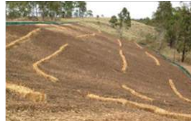
Photo: Erosion control to cleared batter
