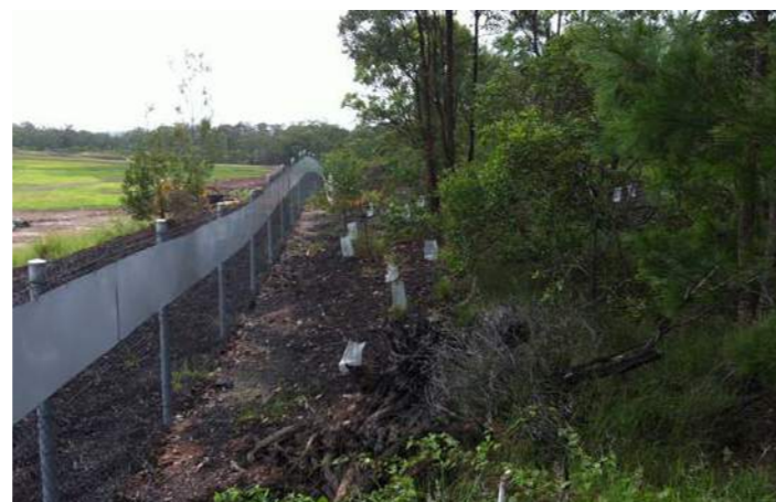
Fauna Exclusion Fencing
