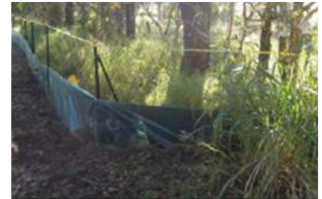
Photo: Tree protection and erosion fence
