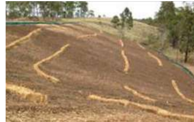
Photo: Erosion control to cleared batter
