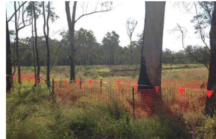
Significant Tree Protection Fencing
