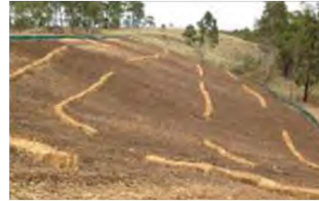
Photo: Erosion control to cleared batter
