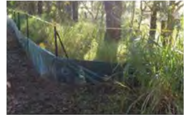
Photo: Tree protection and erosion fence
