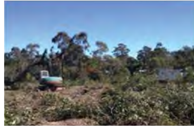
Photo: Control clearing of vegetation
