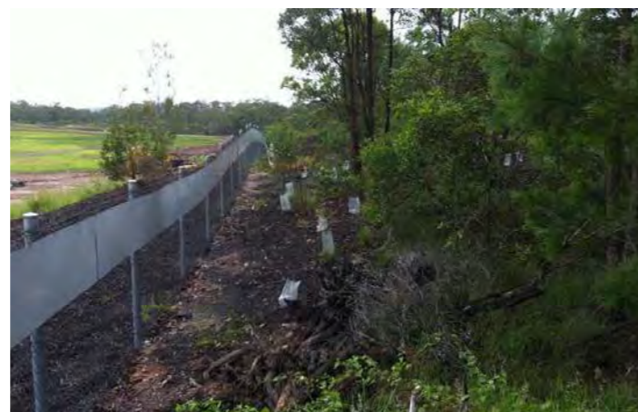
Fauna Exclusion Fencing
