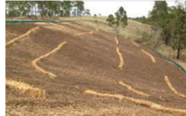
Photo: Erosion control to cleared batter
