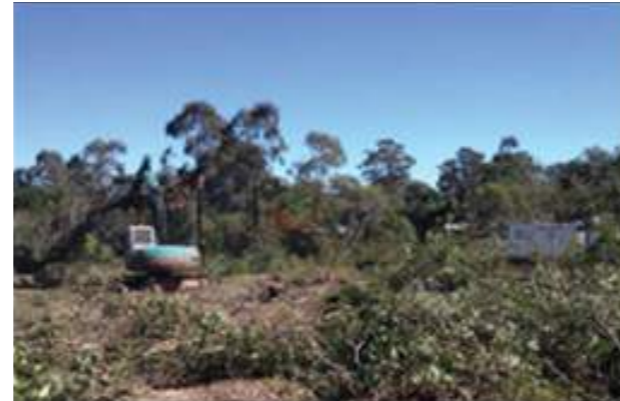
Photo: Control clearing of vegetation
