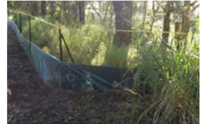
Photo: Tree protection and erosion fence
