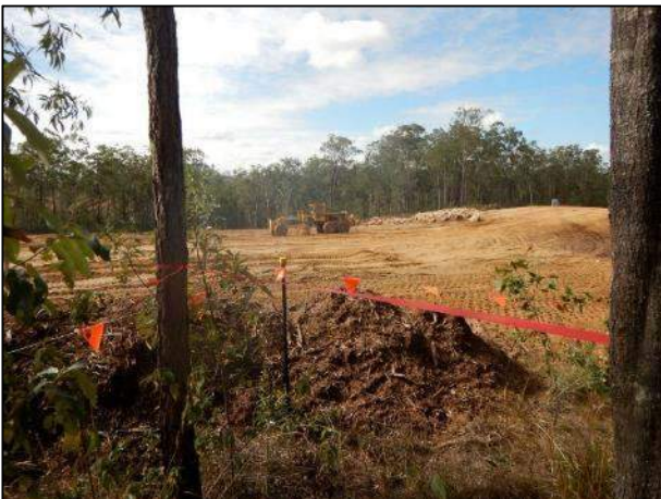
Photo 4: Clearing area within demarcated limits
