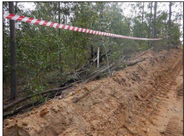
Photo 5: Clearing area boundary
