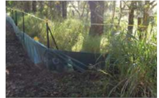
Photo: Tree protection and erosion fence
