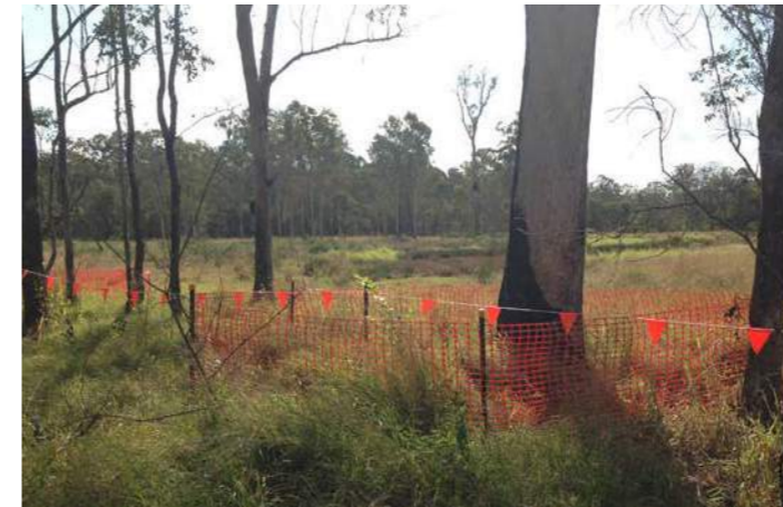
Significant Tree Protection Fencing
