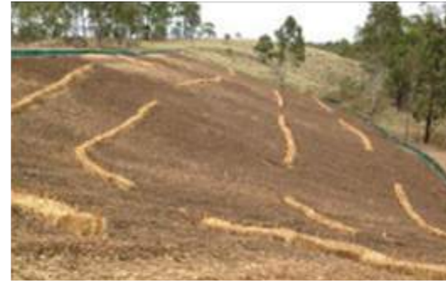
Photo: Erosion control to cleared batter
