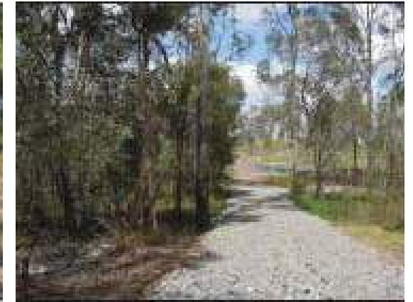
Controlled clearing access track
