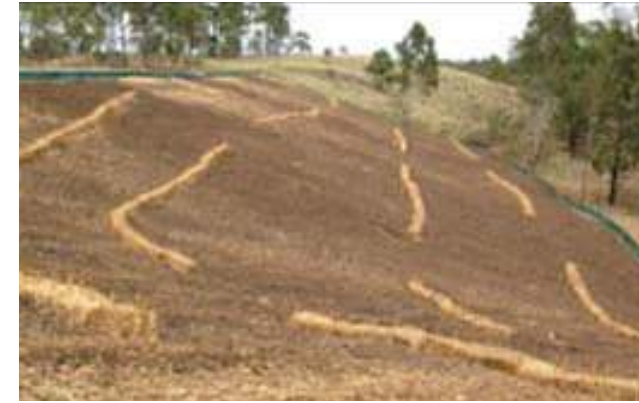
Photo: Erosion control to cleared batter
