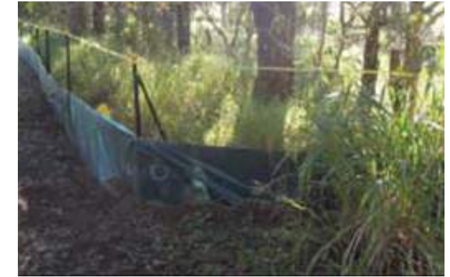
Photo: Tree protection and erosion fence
