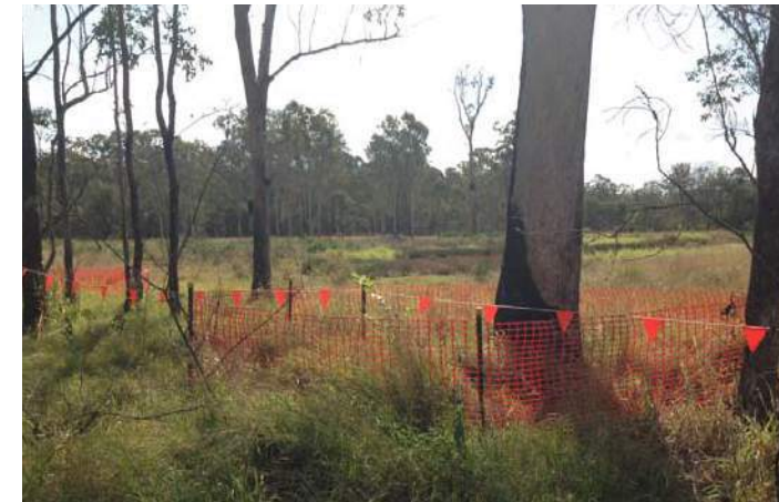
Significant Tree Protection Fencing
