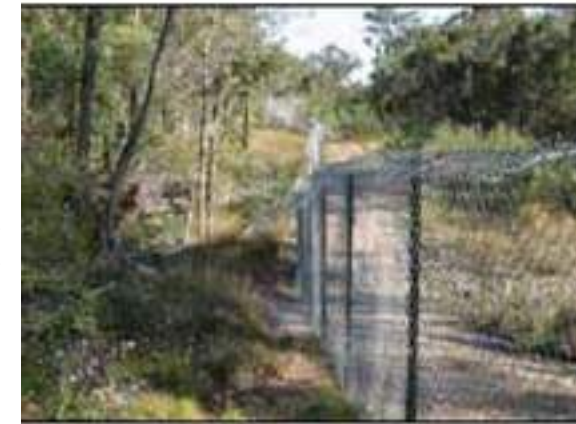
Fauna exclusion fencing
