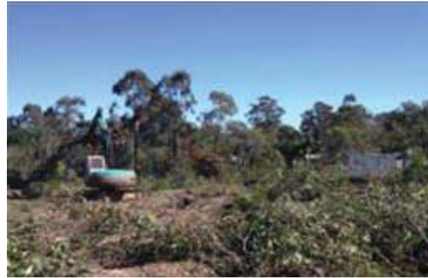
Photo: Control clearing of vegetation
