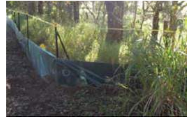
Photo: Tree protection and erosion fence
