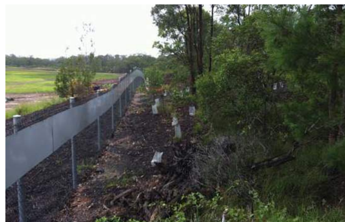
Fauna Exclusion Fencing
