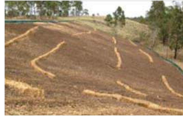
Photo: Erosion control to cleared batter
