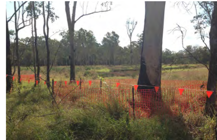
Significant Tree Protection Fencing
