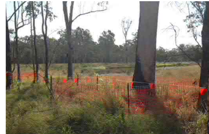
Significant Tree Protection Fencing
