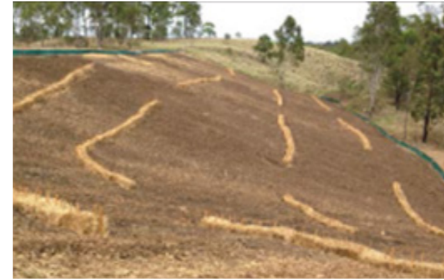
Photo: Erosion control to cleared batter
