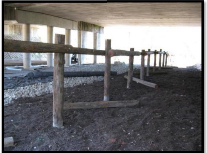
Below – Timber Koala “bridge” forms part of a suite of fauna “furniture” treatments under the Gateway Motorway (Rochedale, Brisbane).
