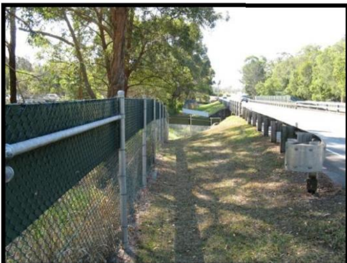
Below - Koala exclusion fencing applied to roadside and bridging over Eprapah Creek (Redland Shire).
