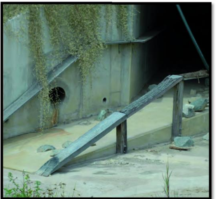
Below – Timber Koala “bridge” forms part of a retrofit to a box culvert under Compton Road, Kuraby (Queensland Government 2009).
