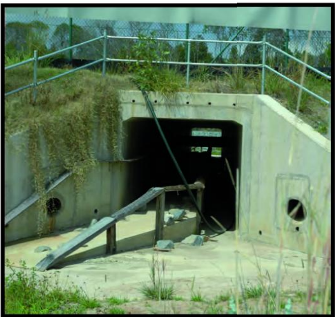
Below – Timber Koala “bridge” forms part of a retrofit to a box culvert under Compton Road, Kuraby (Queensland Government 2009).
