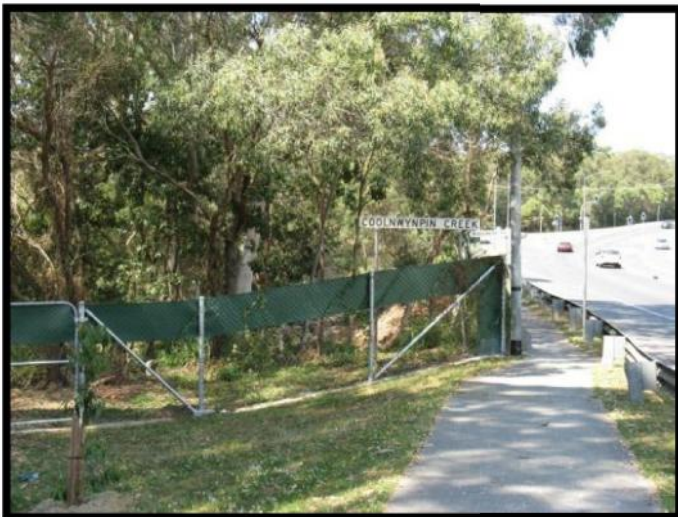
Below - Koala exclusion fencing applied to roadside and bridging over Eprapah Creek (Redland Shire).
