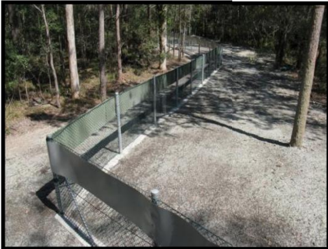
Above - Roadside Koala exclusion fencing with concrete footing (Burbank, Brisbane). Note vegetation management treatments. Below – Koala exclusion fencing applied to roadside and bridging over Coolnwynpin Creek (Redland Shire).
