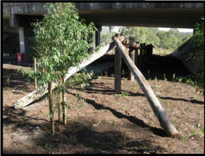
Below – Timber Koala “bridge” forms part of a suite of fauna “furniture” treatments under the Gateway Motorway (Rochedale, Brisbane).
