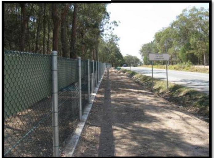
Above - Roadside Koala exclusion fencing with concrete footing (Burbank, Brisbane). Note vegetation management treatments. Below – Koala exclusion fencing applied to roadside and bridging over Coolnwynpin Creek (Redland Shire).
