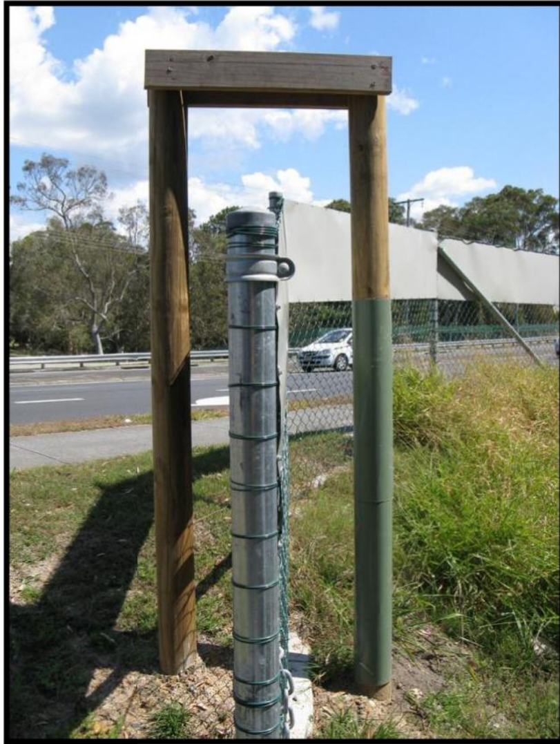
Above – Example of a single-way travel climbing pole (Redland Shire). Colorbond metal collar (on right) prevents the Koala from climbing over fence into the road space, though plain timber pole (left) allows a Koala to escape from the road environment. Below – Examples of climbing poles (Queensland Government 2009).
