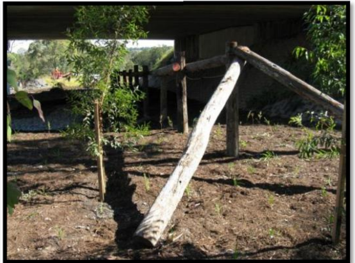
Below – Timber Koala “bridge” forms part of a retrofit to a box culvert under Compton Road, Kuraby (Queensland Government 2009).
