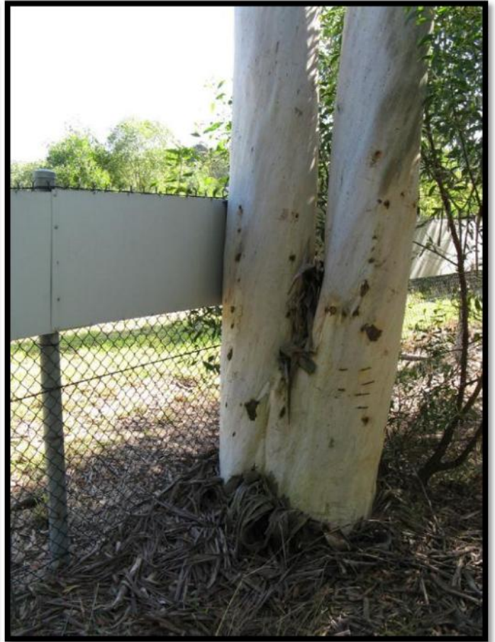
Above & Below – Examples of Koala exclusion fencing functionality being compromised by poor siting and vegetation management (Brisbane).
