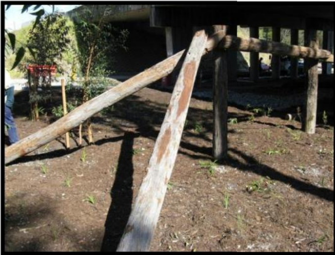
Below – Timber Koala “bridge” forms part of a retrofit to a box culvert under Compton Road, Kuraby (Queensland Government 2009).
