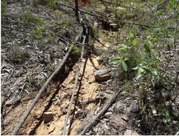
Figure 9: Drainage feature caused by water runoff
