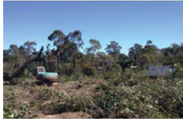
Photo: Control clearing of vegetation
