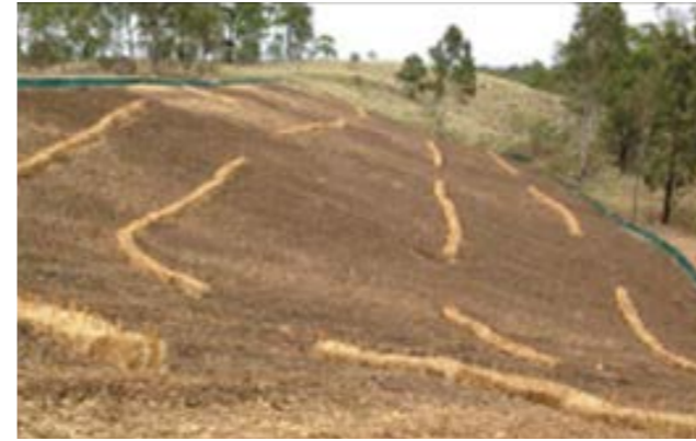
Photo: Erosion control to cleared batter
