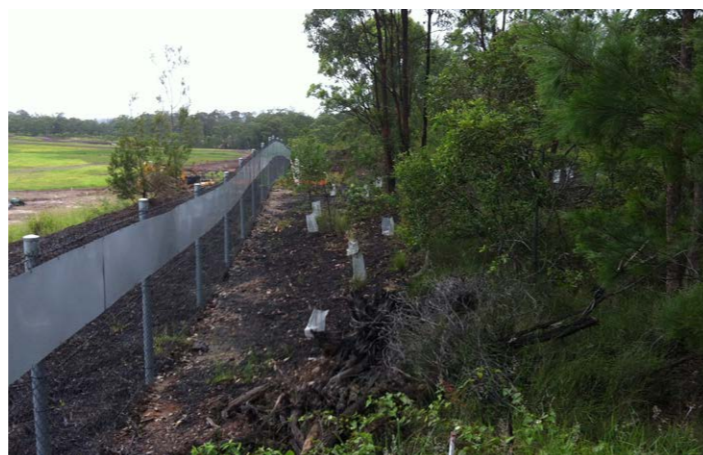
Fauna Exclusion Fencing
