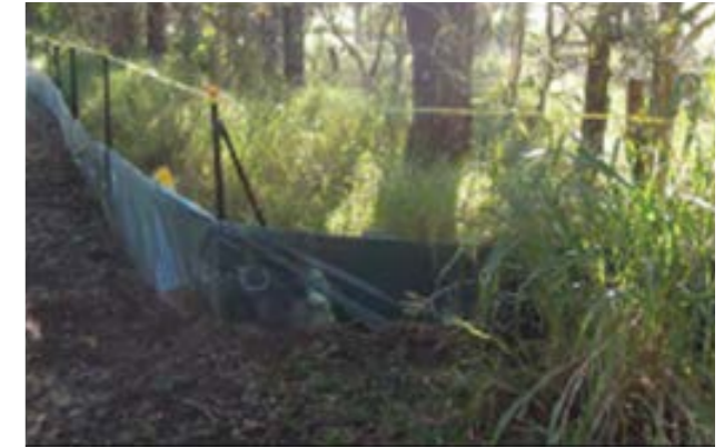
Photo: Tree protection and erosion fence
