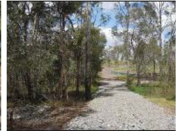
Controlled clearing access track
