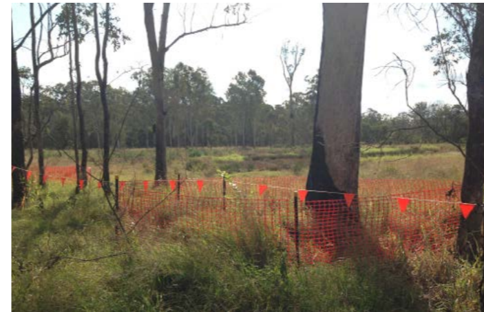
Significant Tree Protection Fencing
