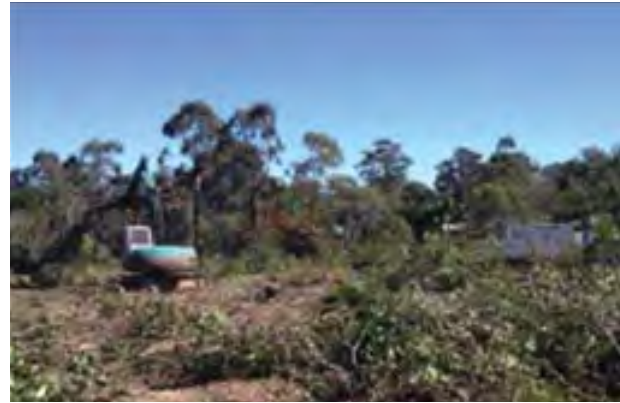
Photo: Control clearing of vegetation
