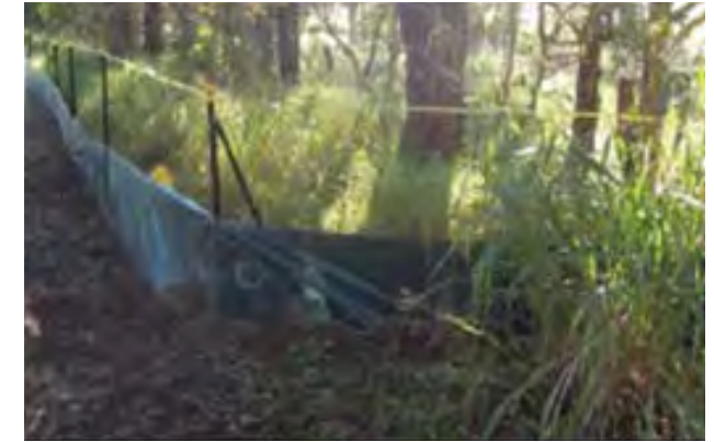
Photo: Tree protection and erosion fence
