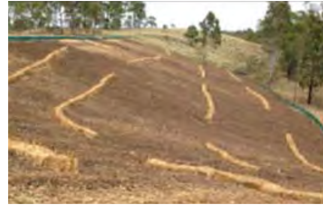
Photo: Erosion control to cleared batter
