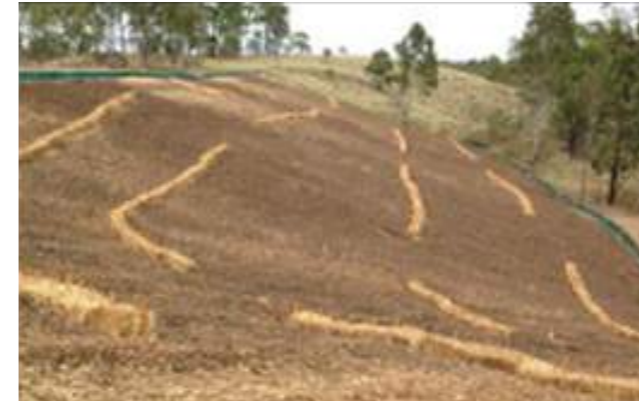
Photo: Erosion control to cleared batter
