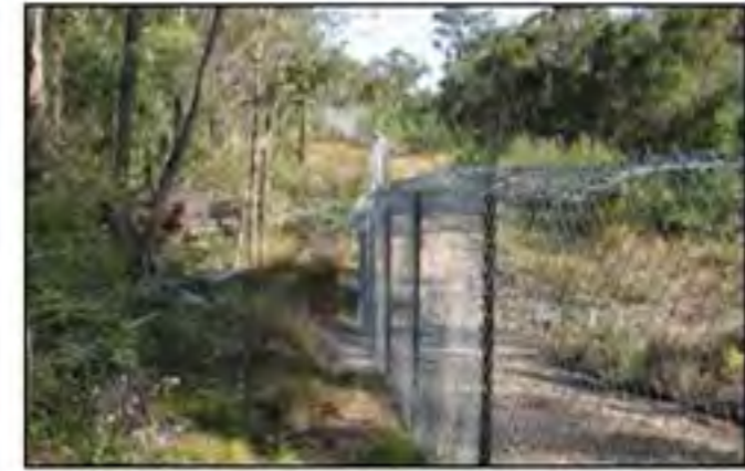
Fauna exclusion fencing
