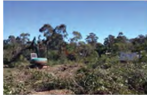
Photo: Control clearing of vegetation
