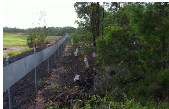
Fauna Exclusion Fencing
