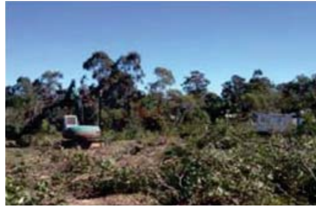
Photo: Control clearing of vegetation
