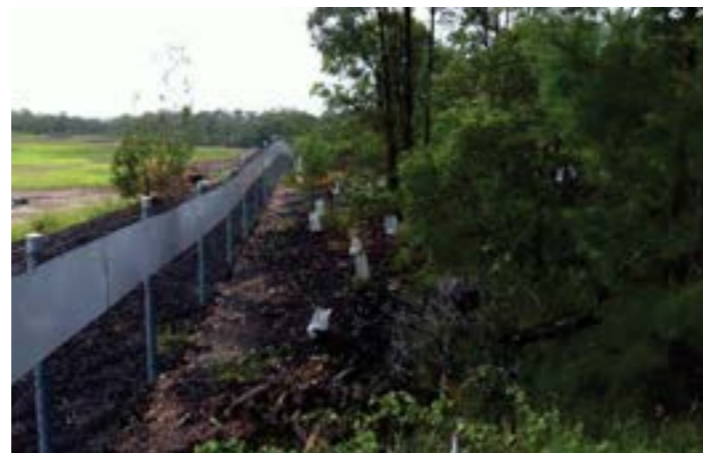
Fauna Exclusion Fencing
