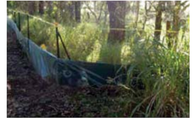
Photo: Tree protection and erosion fence
