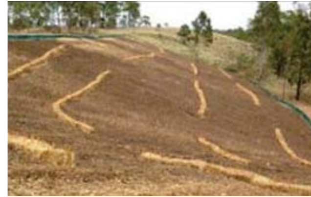
Photo: Erosion control to cleared batter
