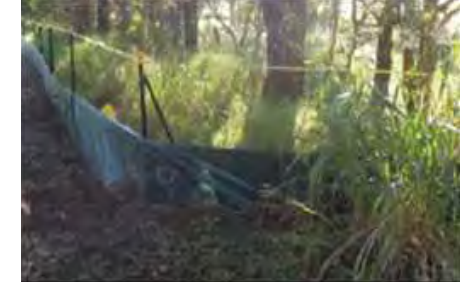
Photo: Tree protection and erosion fence
