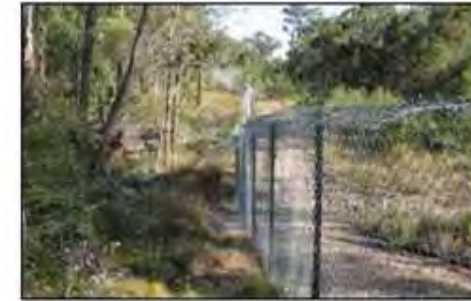
Fauna exclusion fencing
