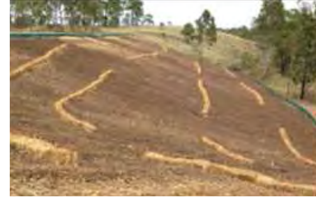
Photo: Erosion control to cleared batter
