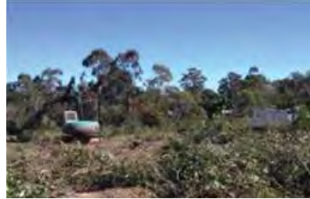
Photo: Control clearing of vegetation
