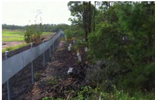
Fauna Exclusion Fencing
