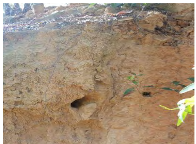
Figure 6: Burrow in embankment
