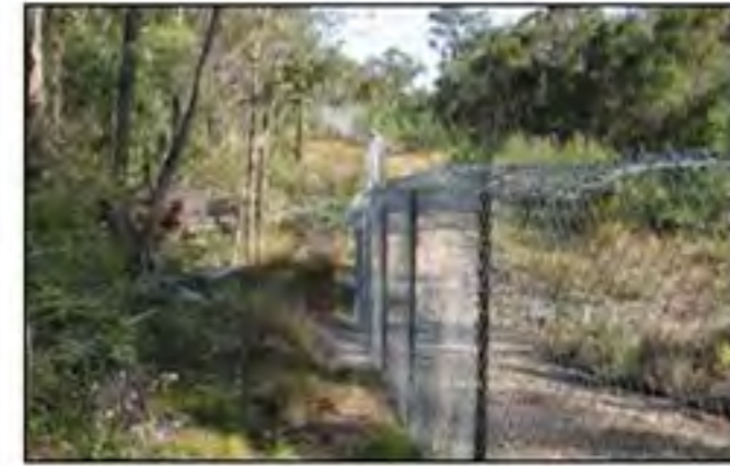
Fauna exclusion fencing
