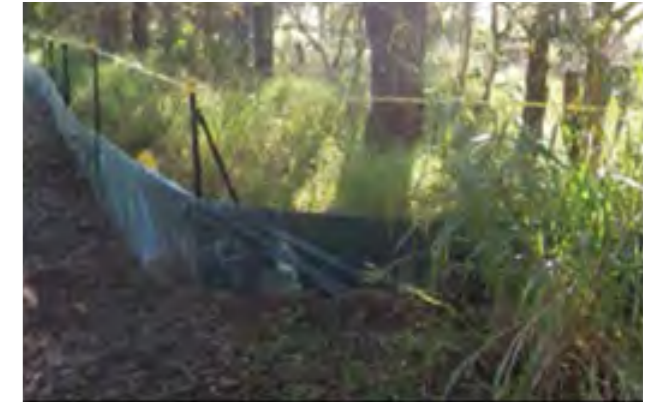
Photo: Tree protection and erosion fence
