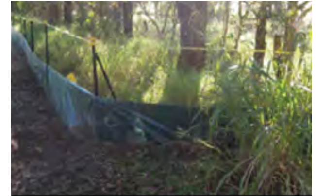
Photo: Tree protection and erosion fence
