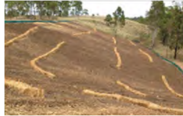
Photo: Erosion control to cleared batter
