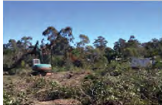
Photo: Control clearing of vegetation
