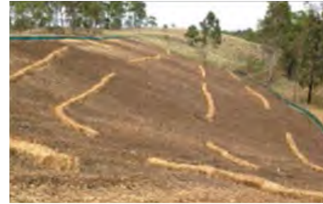
Photo: Erosion control to cleared batter
