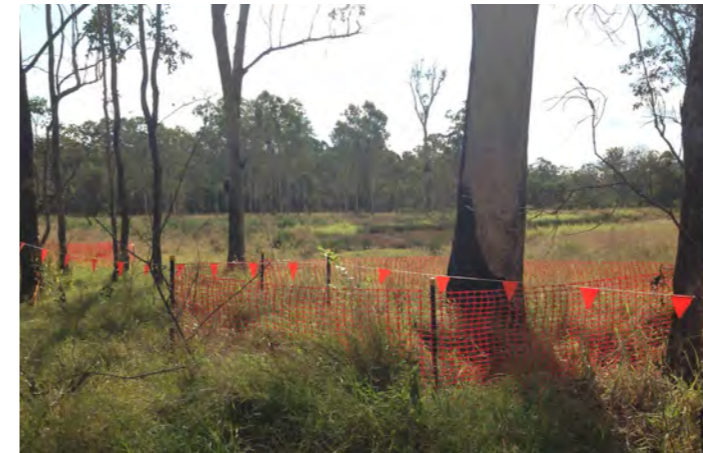
Significant Tree Protection Fencing
