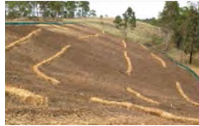
Photo: Erosion control to cleared batter
