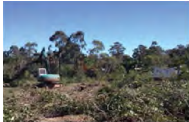
Photo: Control clearing of vegetation
