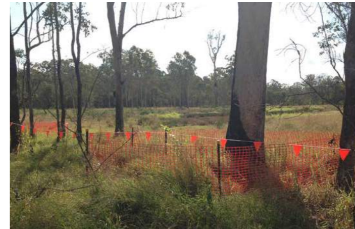
Significant Tree Protection Fencing
