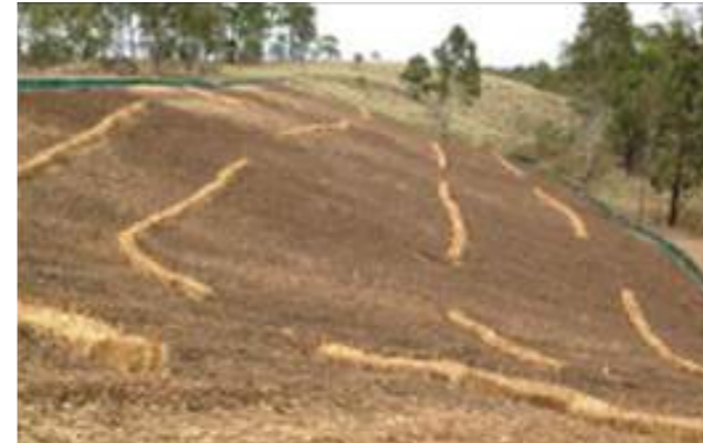
Photo: Erosion control to cleared batter
