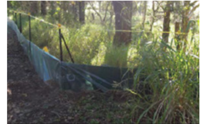
Photo: Tree protection and erosion fence
