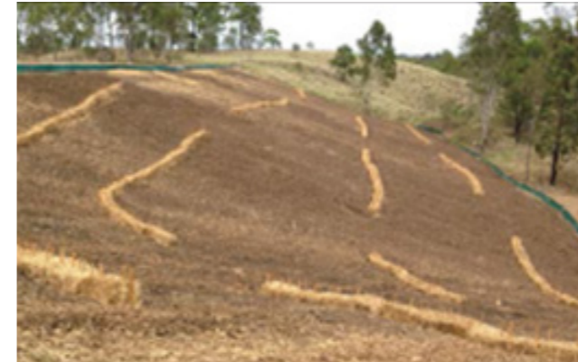
Photo: Erosion control to cleared batter
