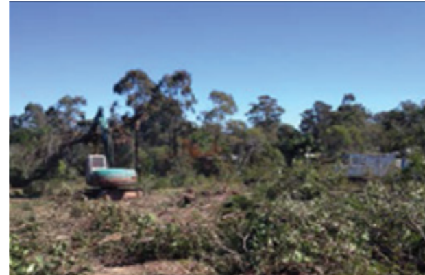
Photo: Control clearing of vegetation
