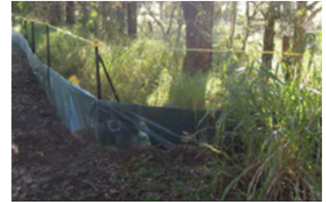
Photo: Tree protection and erosion fence
