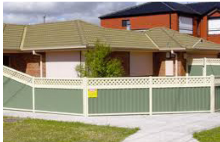
Fauna Exclusion Fencing
