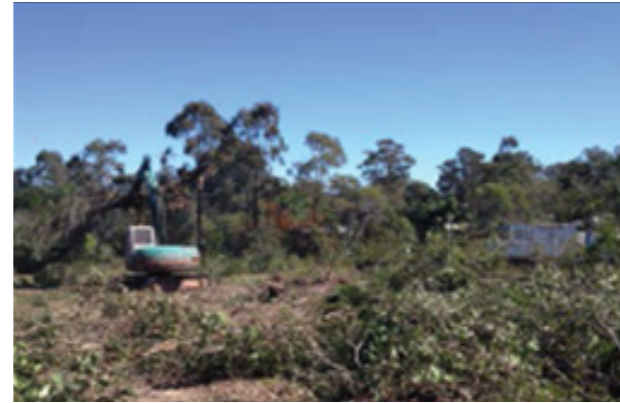
Photo: Control clearing of vegetation
