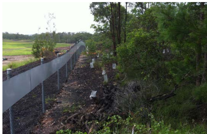
Fauna Exclusion Fencing
