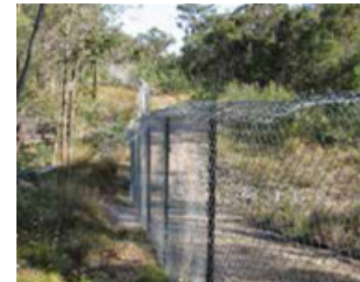
Fauna exclusion fencing
