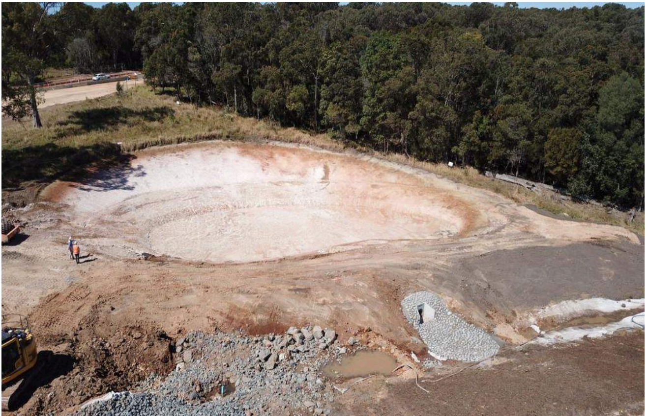
Photo Set 2: Bioretention basin construction
