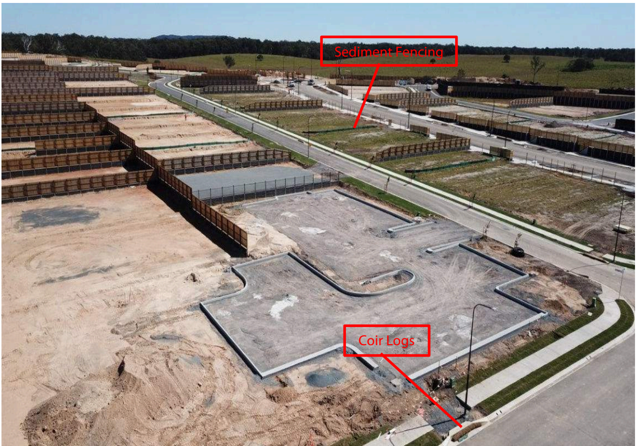
Photo Set 4: Erosion and sediment controls
