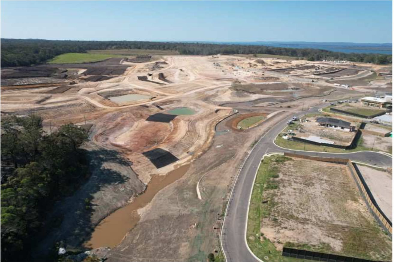
Photo 2: Linear Corridor Overview
