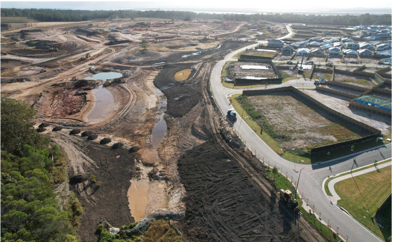
Photo 5: Linear Corridor Overview
