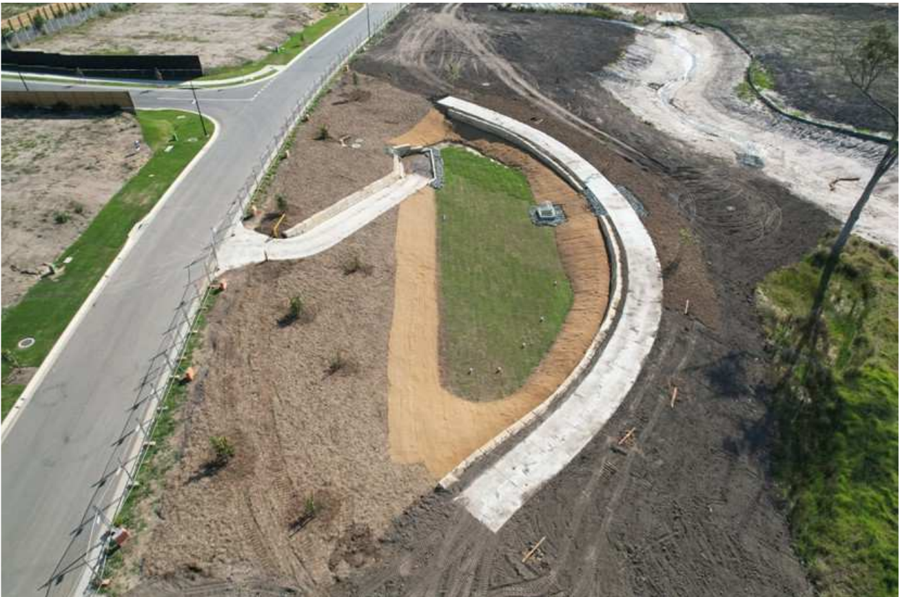
Photo 1: Stage 5 Basin Walls Completion
