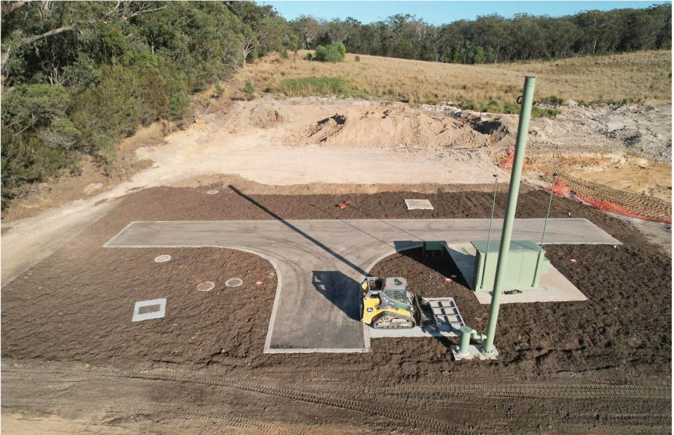
Photo 4: Pump Station Topsoil & Mulch
