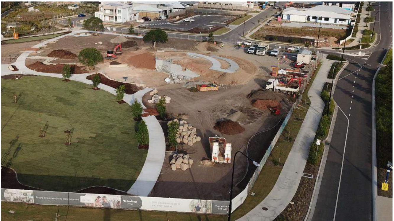
Photo 7: Jingeri park under construction
