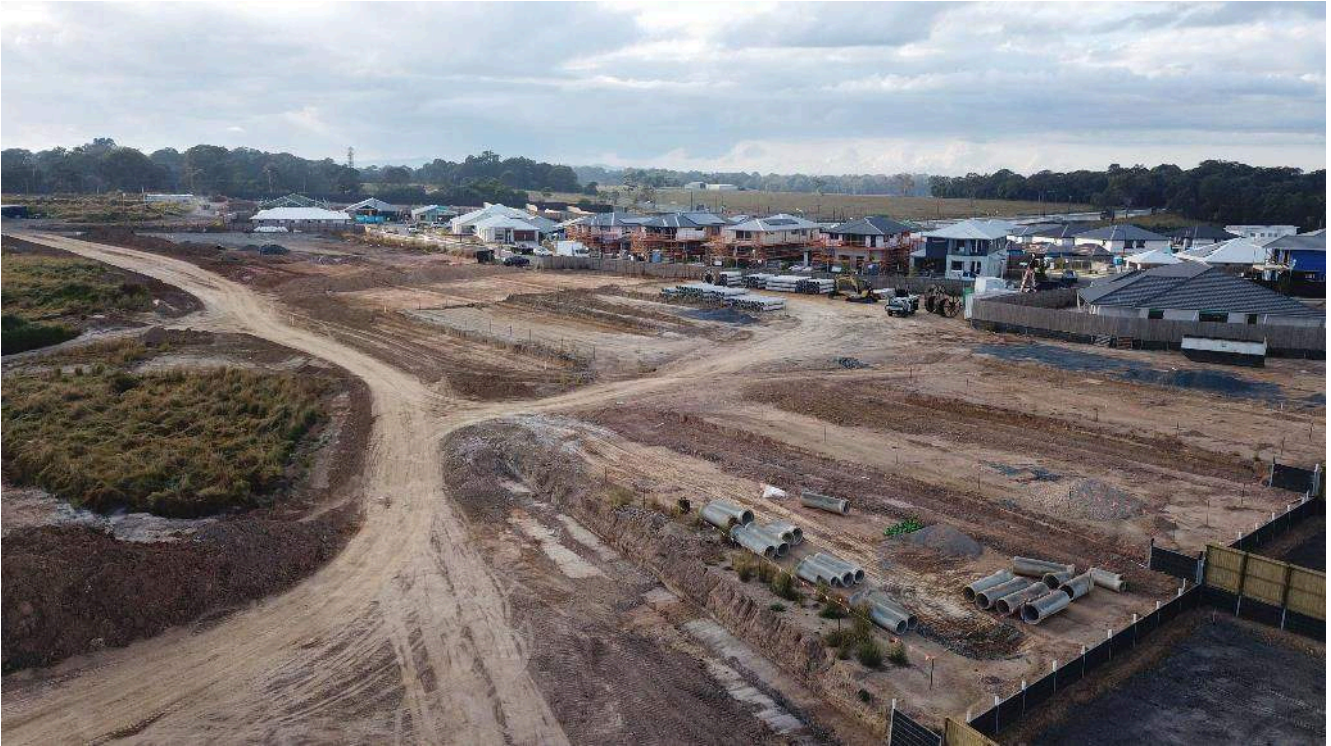
Photo 4: Residential lots and dwelling under construction
