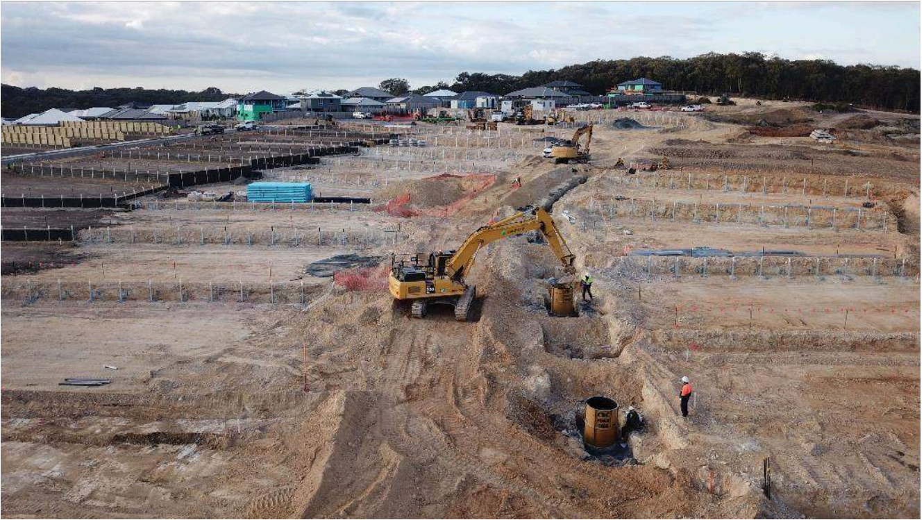
Photo 2: Residential lots under construction
