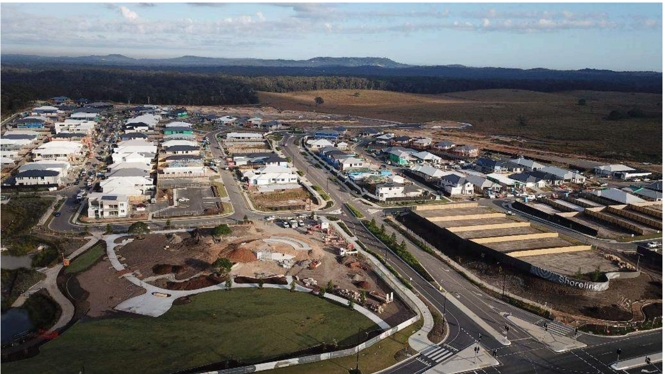
Photo 5: Shoreline main entry alongside established and under construction residential allotments
