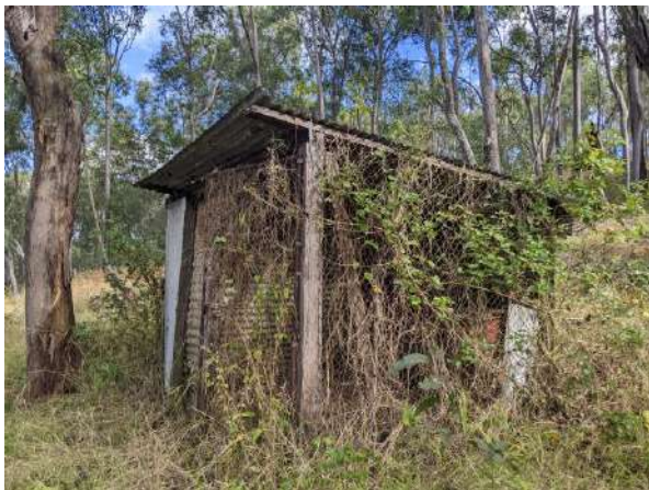
Figure 63: Disused animal enclosure
