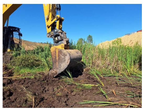
Photo 3 Excavator stripping topsoil
