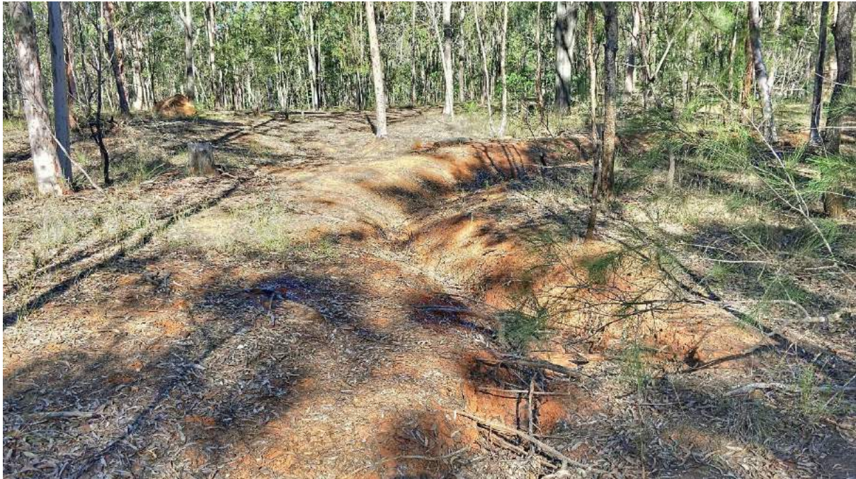
Photo 1: Diversion drain to control erosion on old access track
