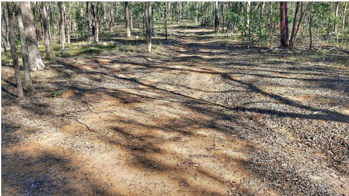
Photo 2: Access Track with Cross Drainage
