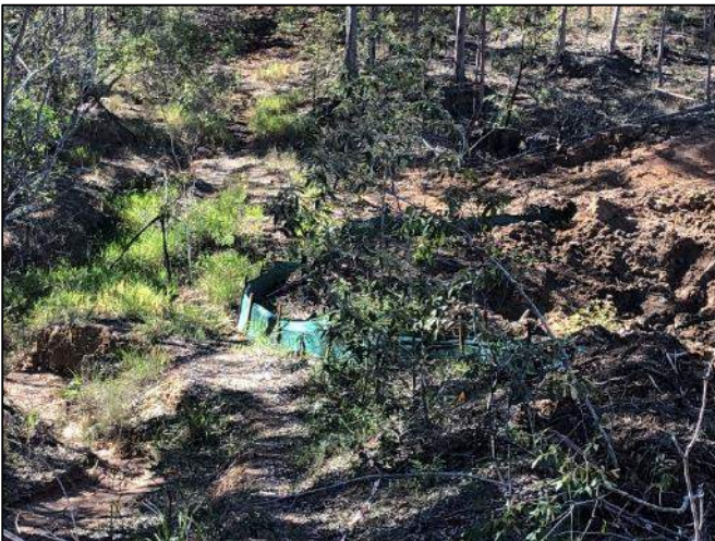
Photo set 5: Sediment control and culverts at Lotus Place bund
