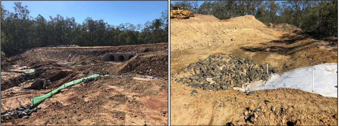
Photo set 10: Earthworks within north-eastern extent of works area
