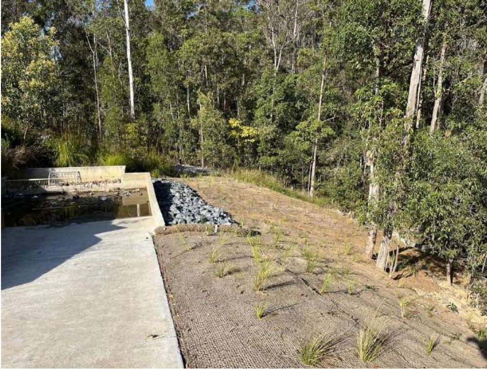
Photo 8: Erosion and sediment controls adjacent an outlet.
