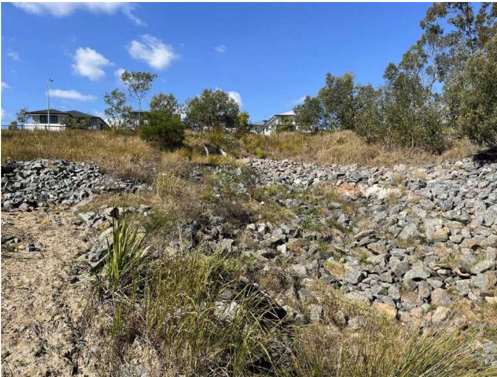
Photo 9: Erosion and sediment controls.
