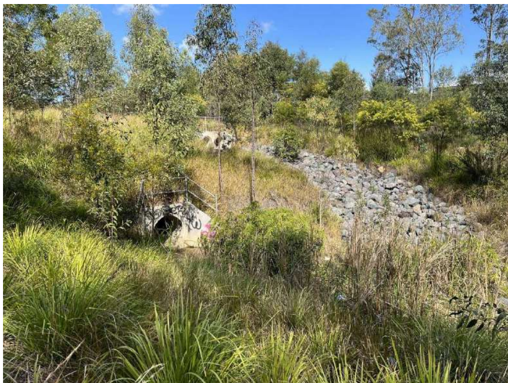
Photo 6: Rehabilitation progressing in the northern drainage interface.
