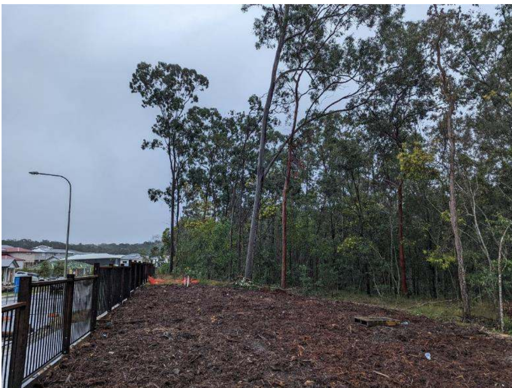
Photo 3: New clearing area with newly installed fence and mulch.
