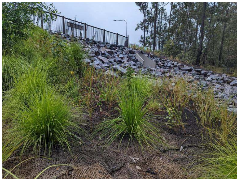
Photo 7: Erosion and sediment controls adjacent an outlet.
