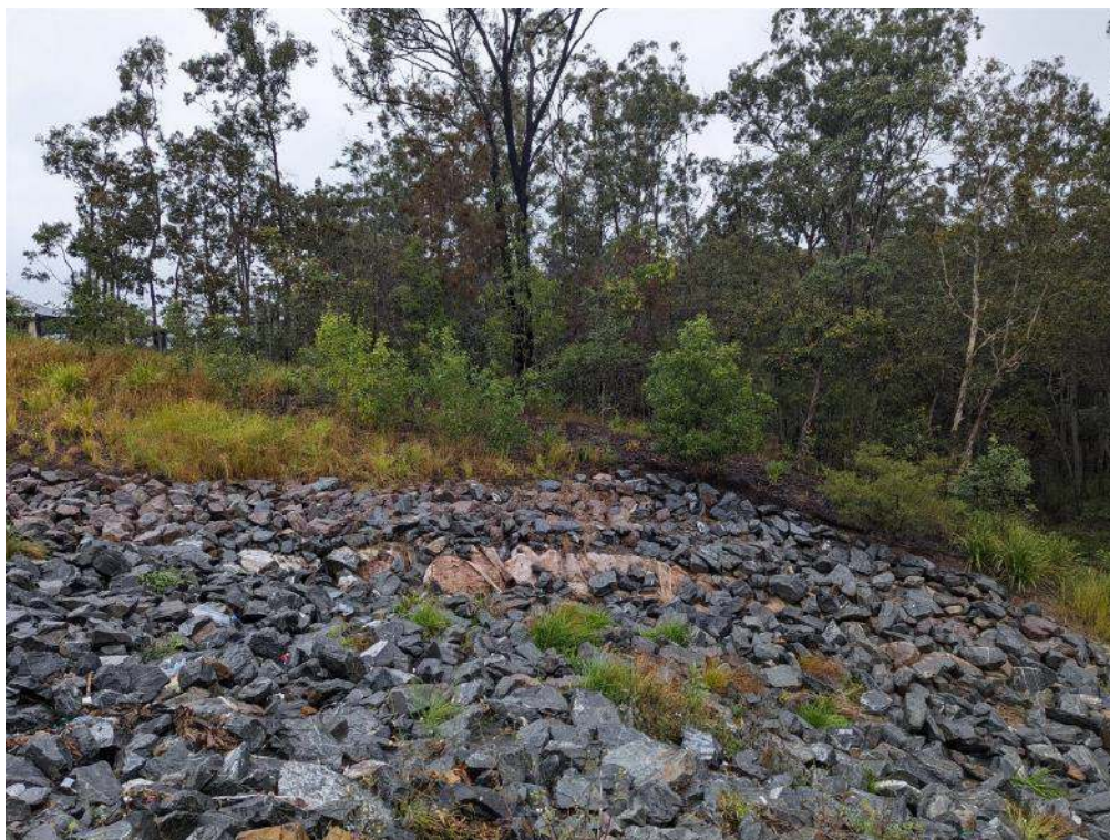
Photo 8: Erosion and sediment controls
