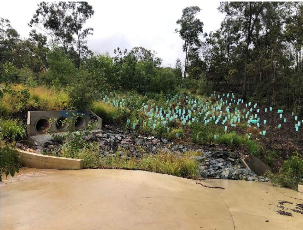
Photo 3: Progress of rehabilitation area at Lotus Place.
