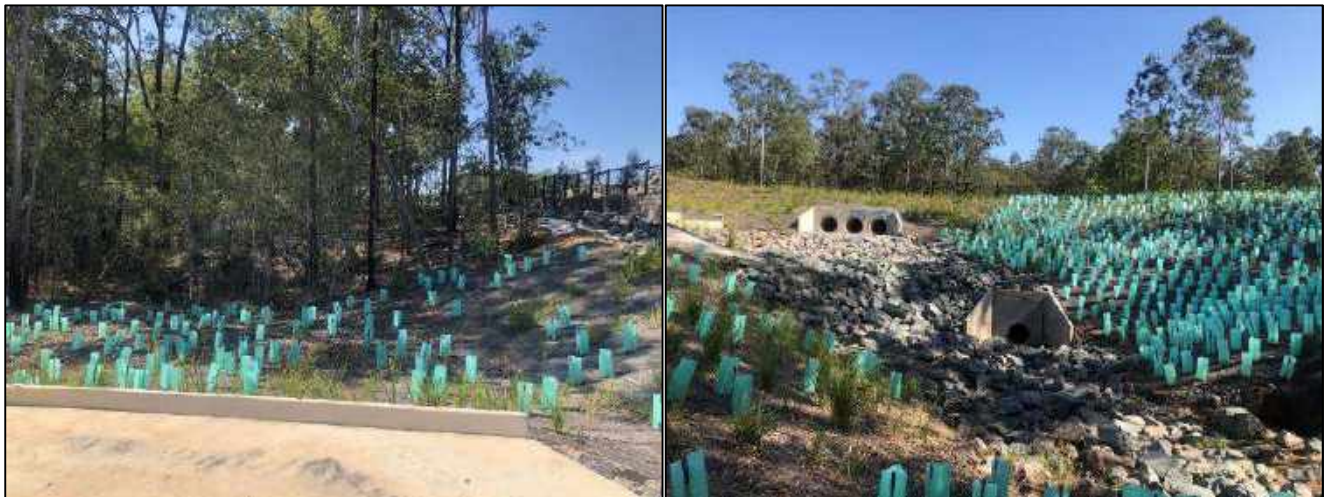
Photo set 7: Rehabilitation works at Lotus Place
