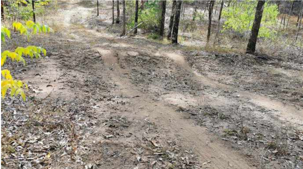
Photo 1: Access Track with Cross Drainage June 2020
