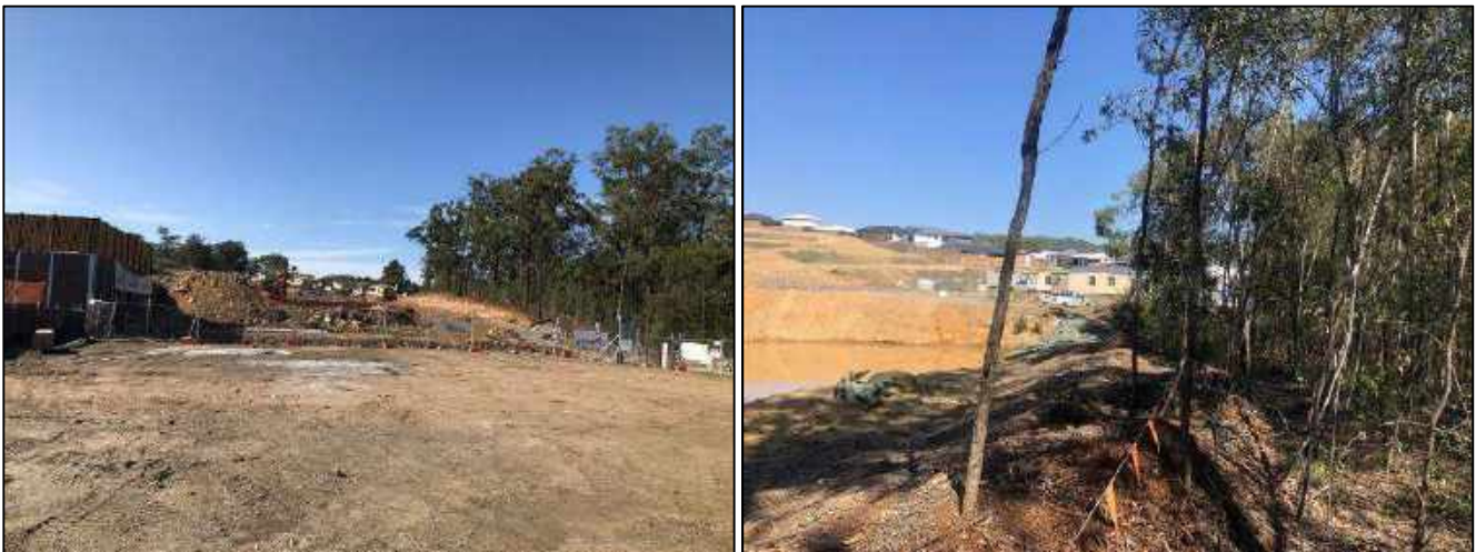
Photo set 5: Associated construction work facilities
