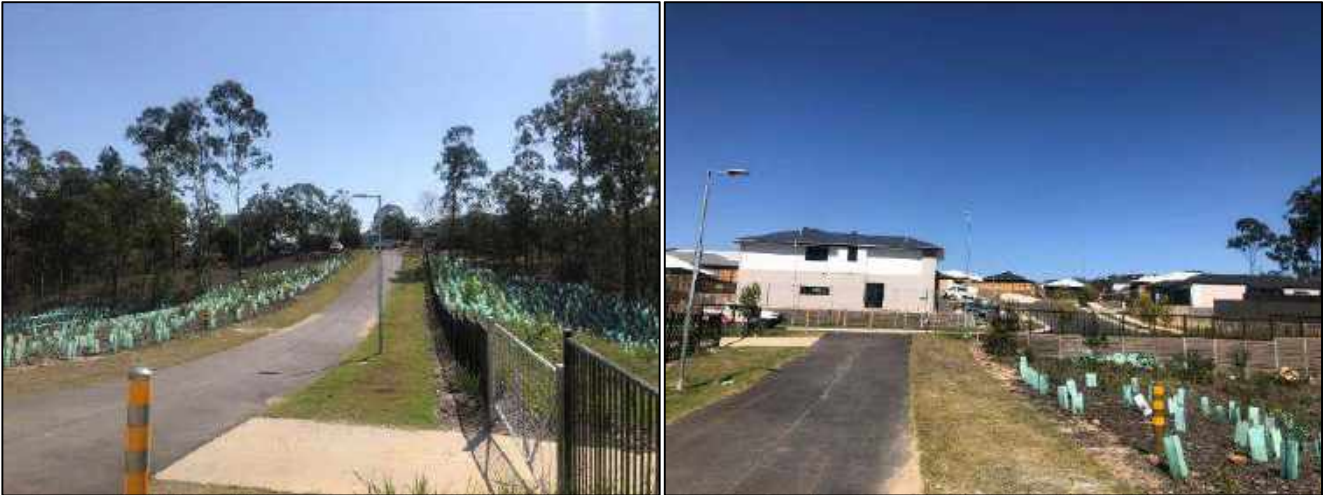
Photo set 6: Rehabilitation works at Lotus Place
