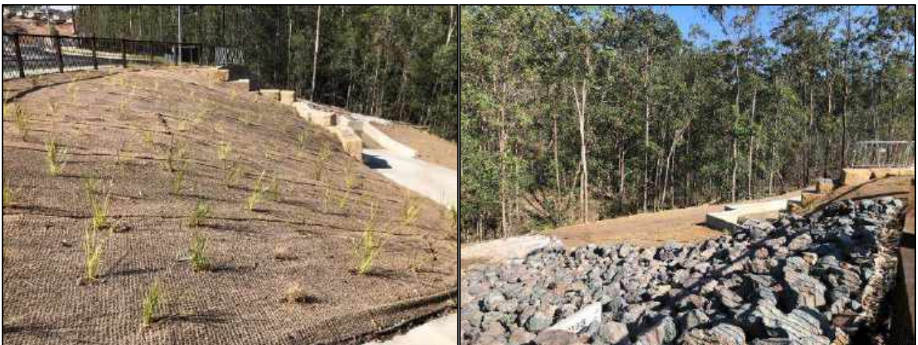
Photo set 8: Erosion and sediment control adjacent to gully line proximal to West Bund
