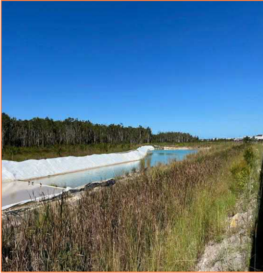
Figure 2-4: High efficiency sediment basins
