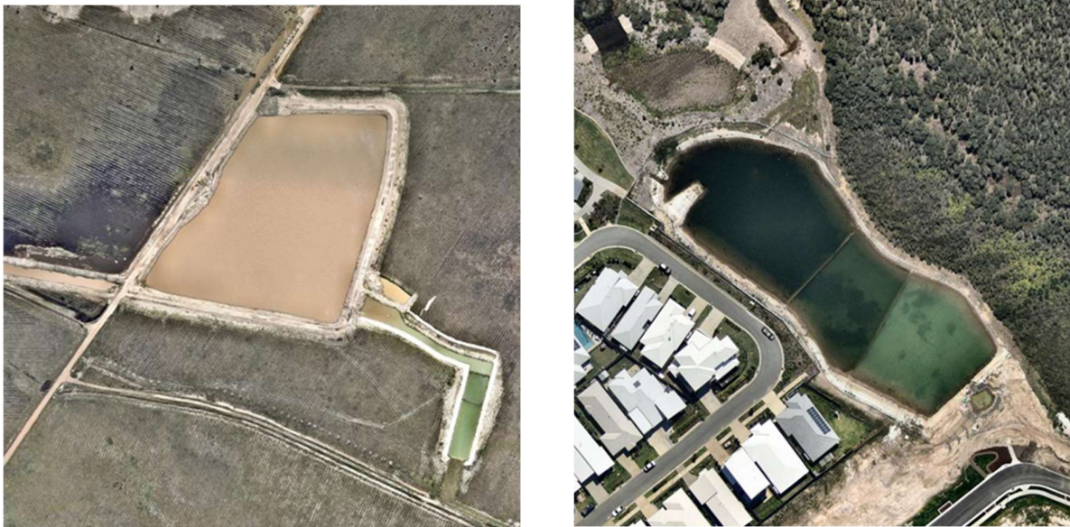
Figure 2-5: Hybrid Sediment Basins in Operation
