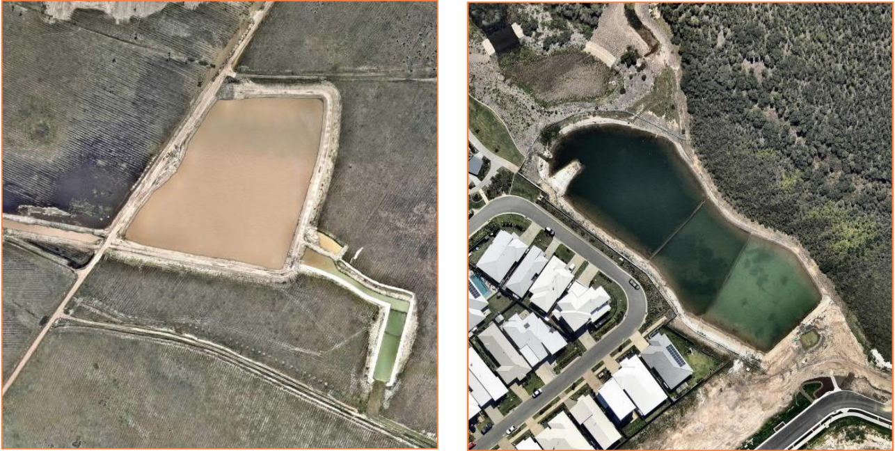
Figure 7: Hybrid Sediment Basins in Operation
