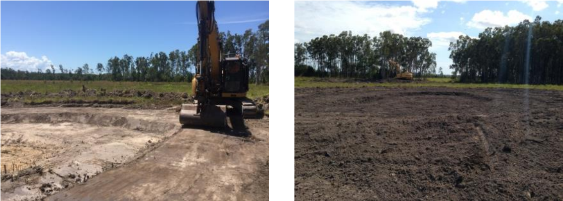
Figure 4: Construction of Wallum Sedge Frog Ponds in Precincts 4 and 5
