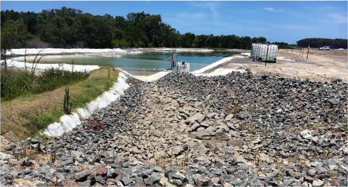
Figure 8: High Efficiency Sediment Basin Installed as Part of Precinct 2 Works
