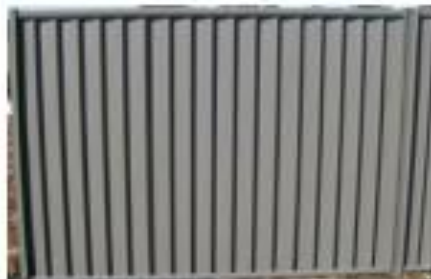
Side and rear boundary fencing
