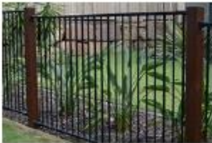
Typical front fencing
