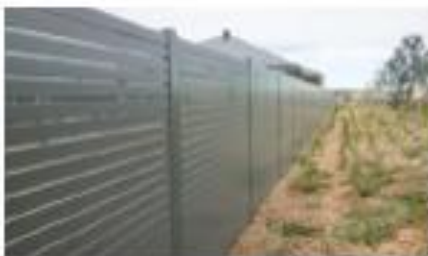
Corner lot fencing
