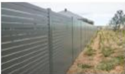
Corner lot fencing
