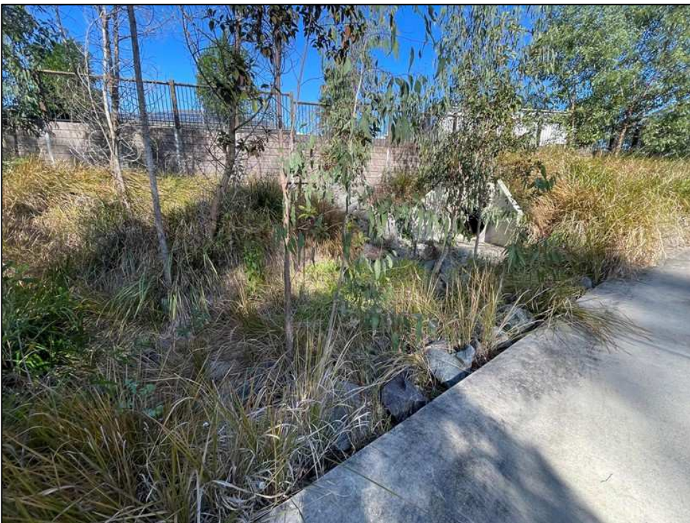
Photo set 3: Rehabilitation Progress of Drainage Area – North-east (Lotus Place)
