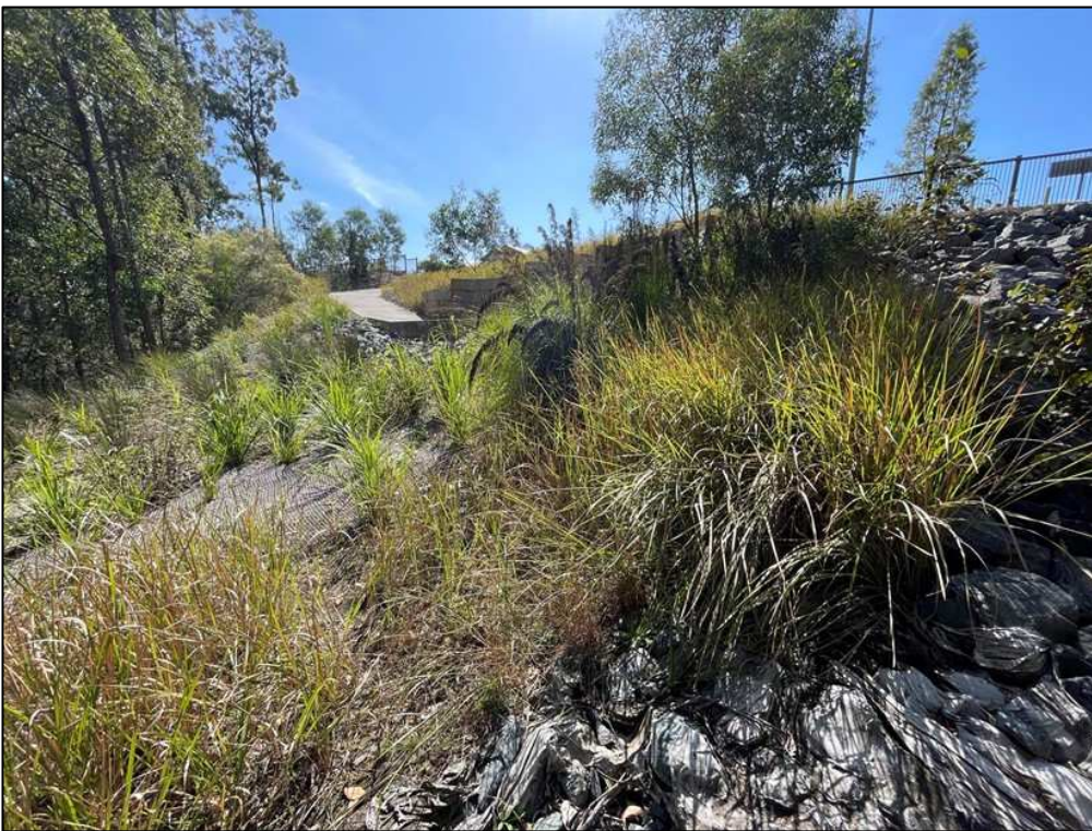
Photo set 5: Rehabilitation Progress of Drainage Area – South-west (Telopea Way)
